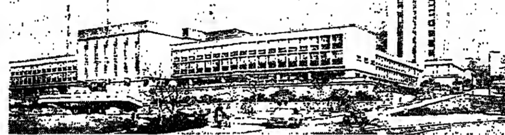
Artist's impression of the £8m Oldham Civic Centre due for completion in early 1978 by Henry Boot Construction. Incorporated will be a council chamber, civic reception area, three-storey multi-purpose assembly hall with service rooms, computer suite, underground car park and office accommodation.
